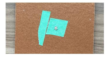
**3.** Peel off the masking tape, and use a razor blade to gently shave off excess filler material until smooth.
